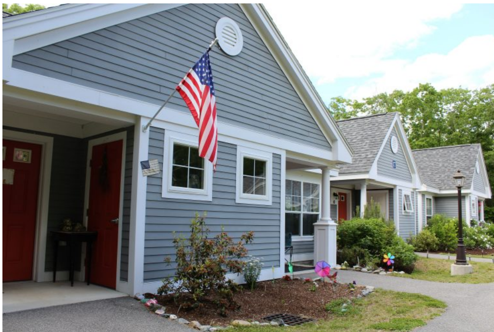
Supportive housing projects such as the Cindy Cookson House in Ellsworth serve as long-term housing for some of Maine’s homeless population. | courtesy of Community Housing of Maine
